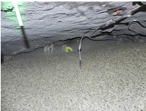
Upper part of the drift – space for backfilling by the spraying
