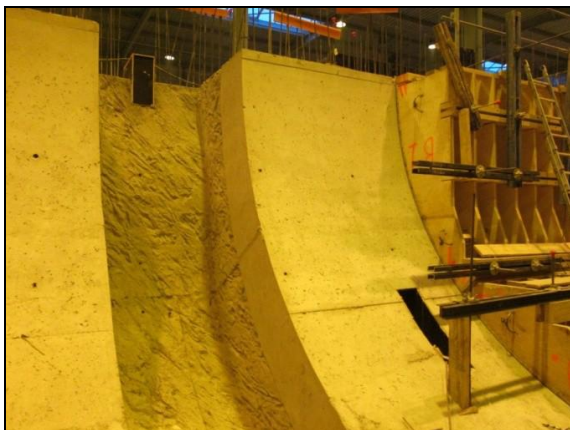
c) the folio pasted on the wood circular inner form to simulate the argillite walls
