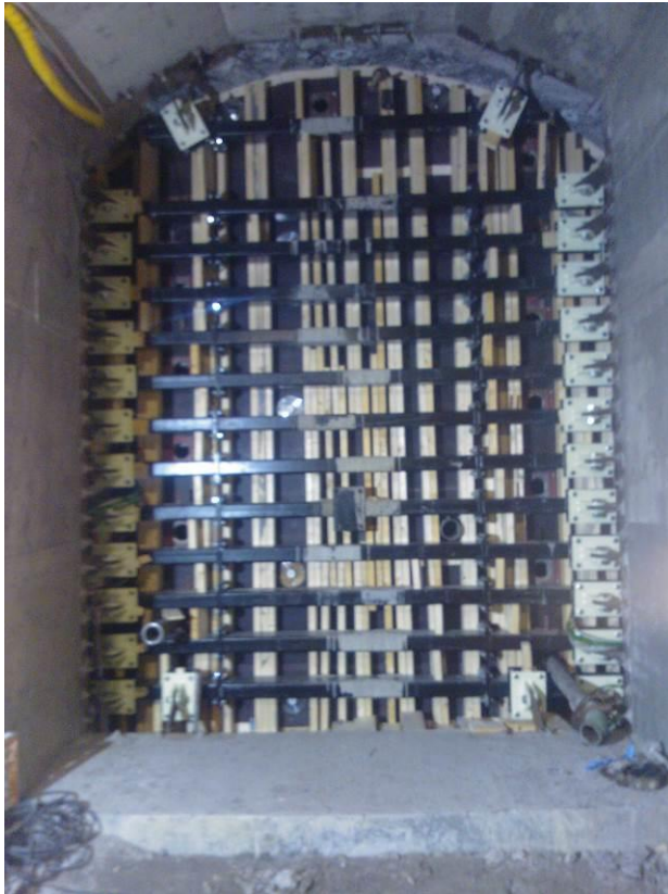
Formwork ready for casting, Concrete Wedge Section One.
