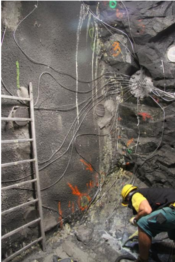
Sensor assembly on inner plug before bentonite emplacement (5.6.2015)
