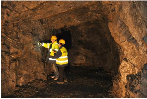
Experimental niche prior to reshaping and ground improvement (2.11.2012)
