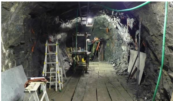
Grouting works
