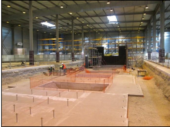
a) View of the concrete foundation
