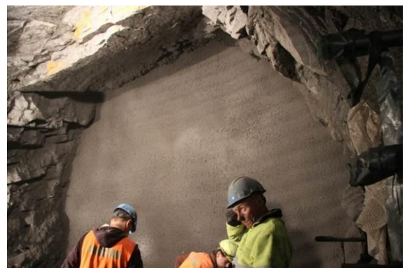
Inner plug erection and sensor installation (12.-13.12.2014)
