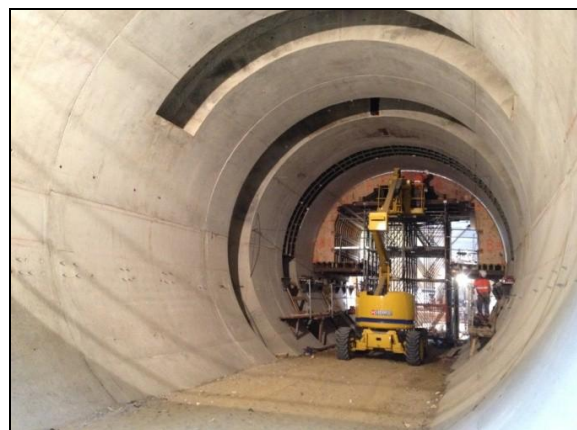
f) The completed test box
