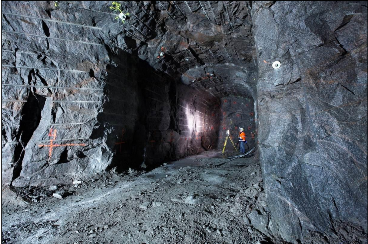
Figure 4.7: The fully excavated DOMPLU experiment tunnel.
