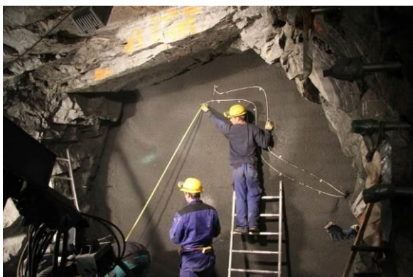
Inner plug erection and sensor installation (12.-13.12.2014)
