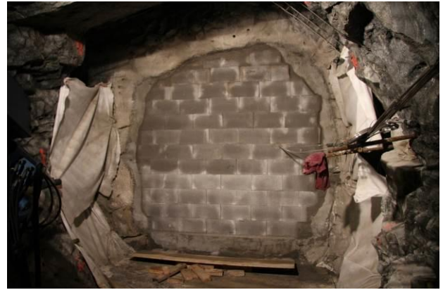
Finished separation wall (5.11.2014)
