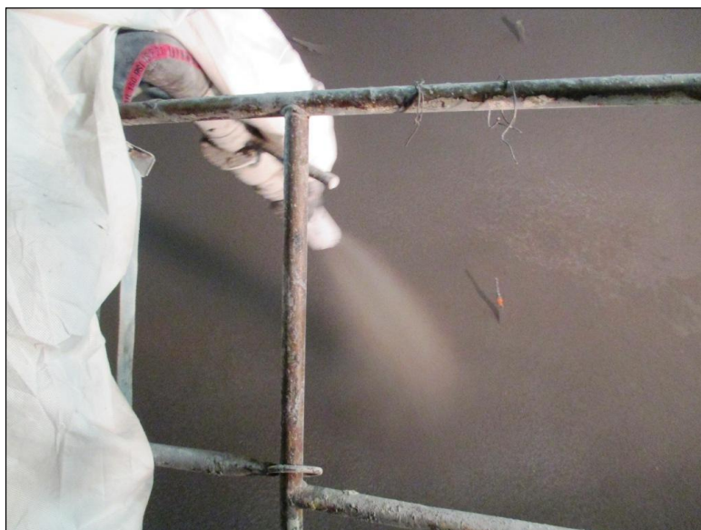
Figure 2.17: Installing the second containment wall made of shotcrete in FSS.
