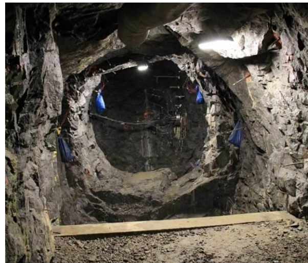
Excavated slots for the plugs
