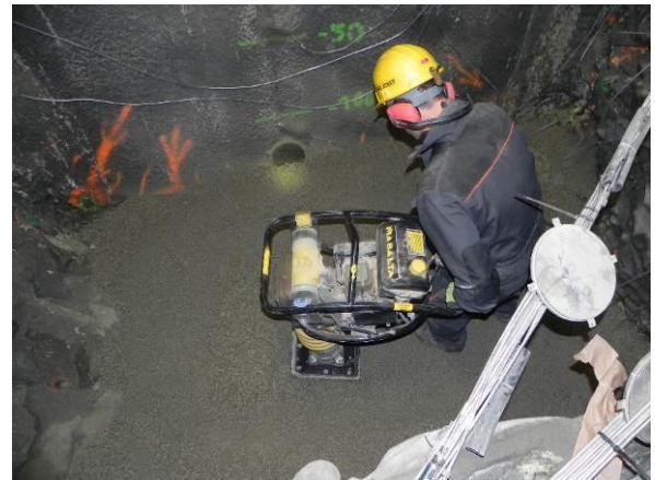
Pellets emplacement (compaction)
