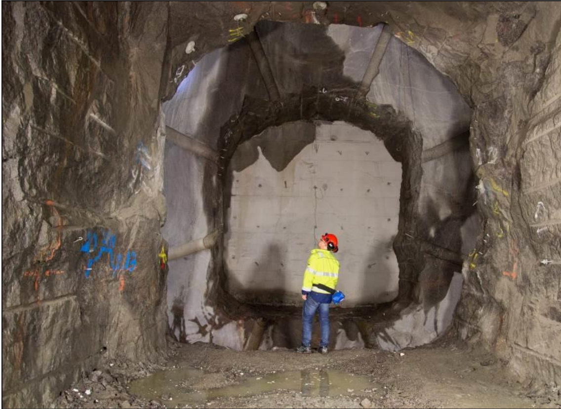
Figure 4.8: The excavated slot abutment for the concrete dome.
