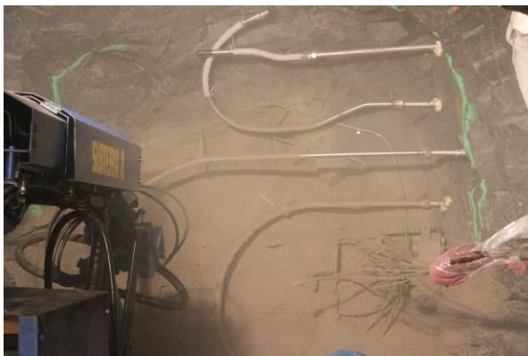
Shotcreting of chamber (27.10.2014)
