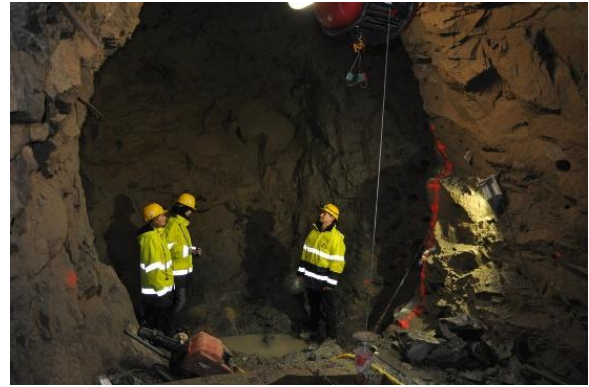
Excavation of slots for plugs
